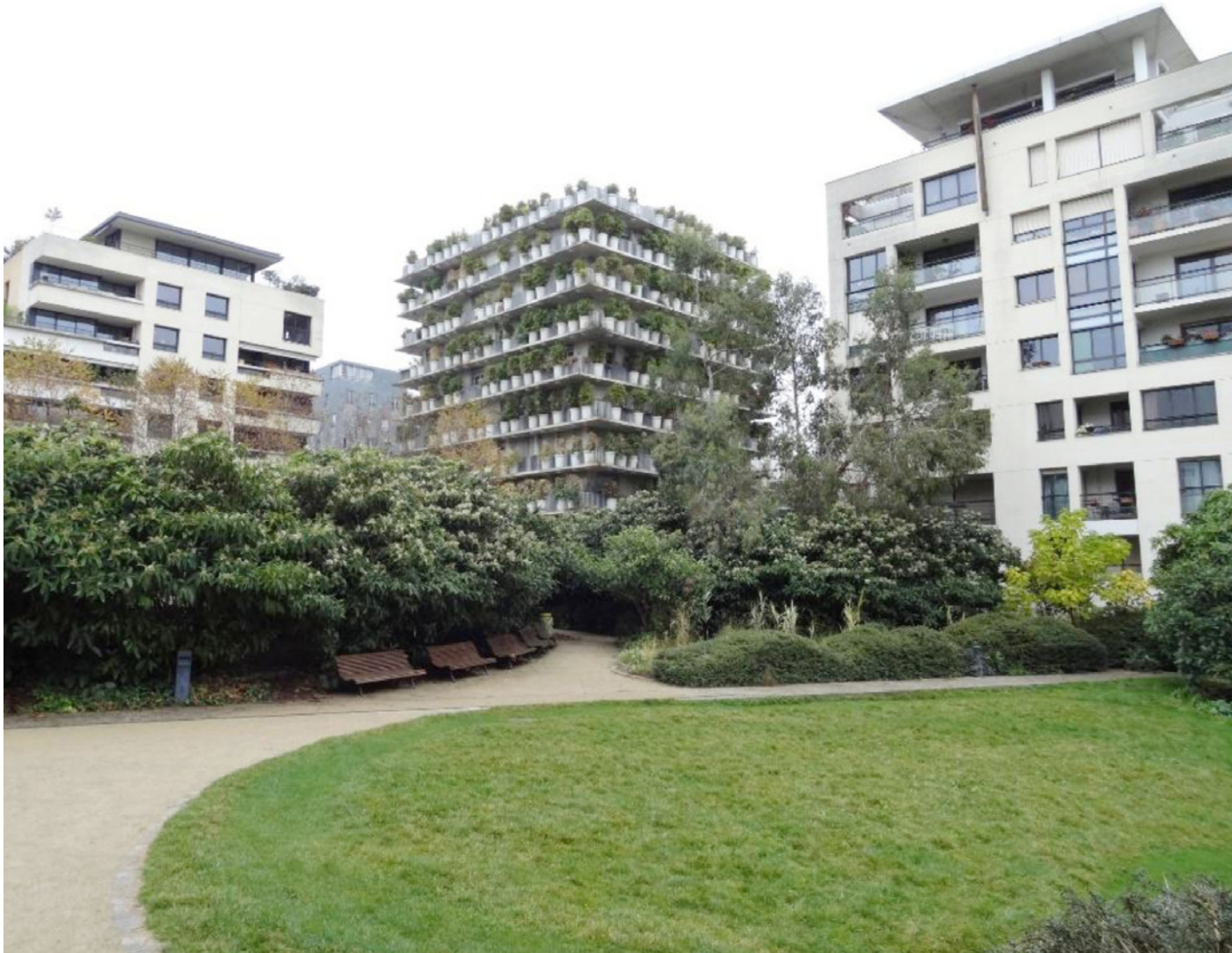
Fig. 4. Flower Tower, Paris - façade details, architect: Eduard Francois; photo: by the author
