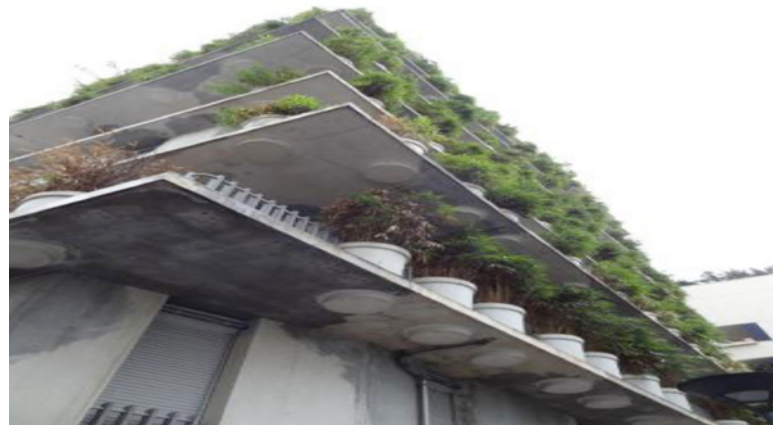
Fig. 5. Flower Tower, Paris, architect: Eduard Francois. Façade details; photo: by the author
