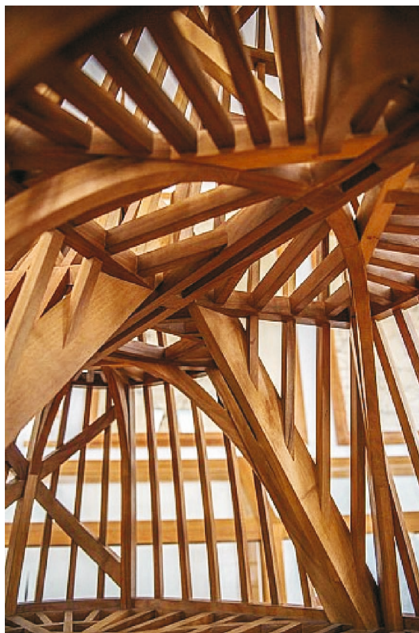
Fig. 4. a, b, c, d. Contemporary wooden architectural models crafted using wooden stereotomy; source: Exposition de chefs-d'oeuvre de Compagnons (2002).
