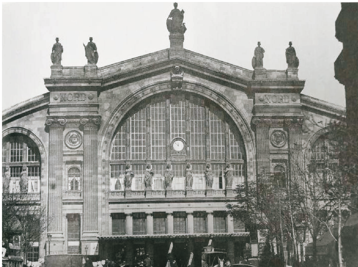
Fig. 10. Paris – Gare du Nord railway station (1861-1865); source: B. Fletcher, A History of Architecture , Architectural Press, London 1996, p. 1127.
