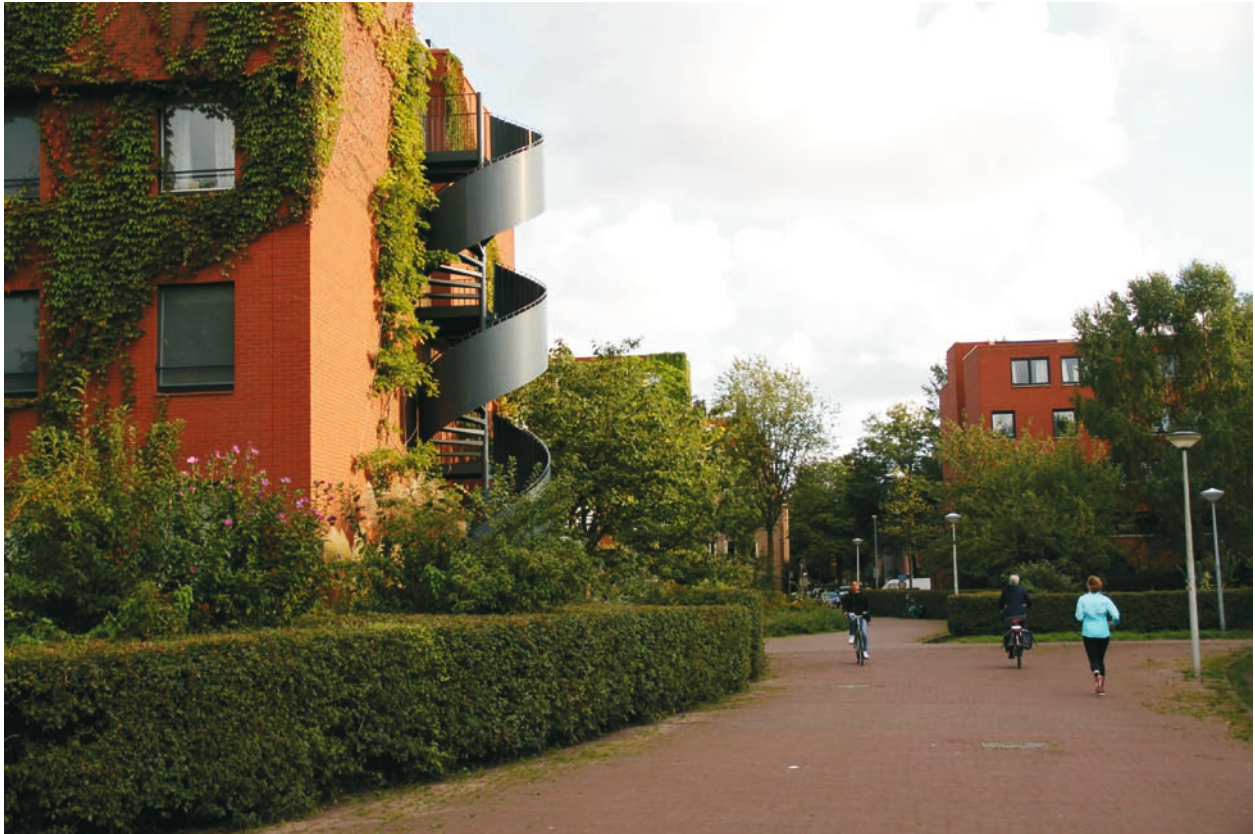
Fig. 4. GWL Terrein, Amsterdam – view of pedestrian and bicycle paths with new buildings and greenery (right); source: photo by the author
