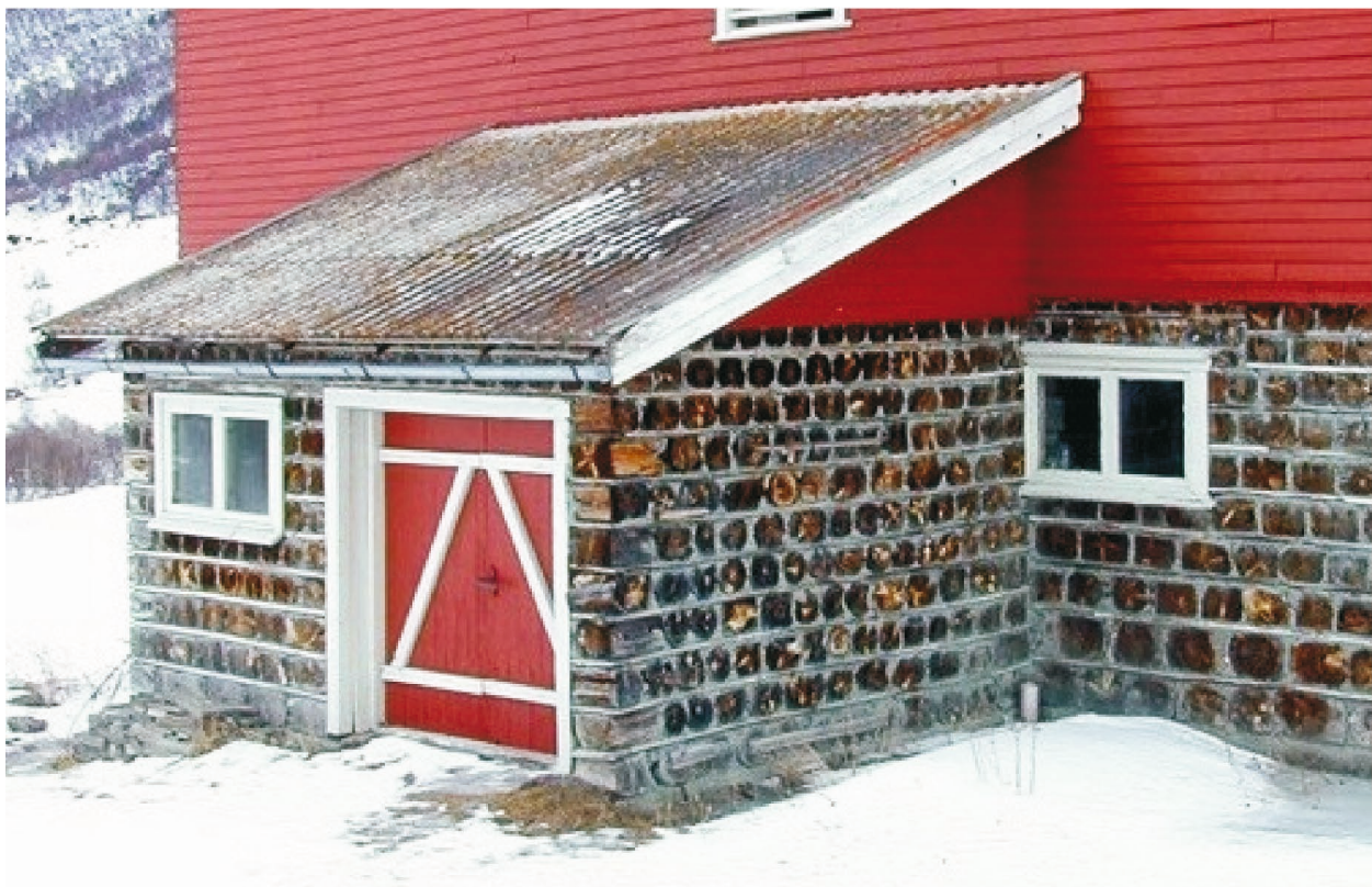
Fig. 3. Barn of cordwood for animal keeping built in the historical period at the farm Risgjerdet in Oppdal in Norway, with logs that are 30 cm long (Stenby, 2021b). The logs seem to be reused from a previous log house, and there are horizontal planks or battens for stability sandwiched in between each layer of logs; photo by: [Hemmingsen & Stensen, 2021]
