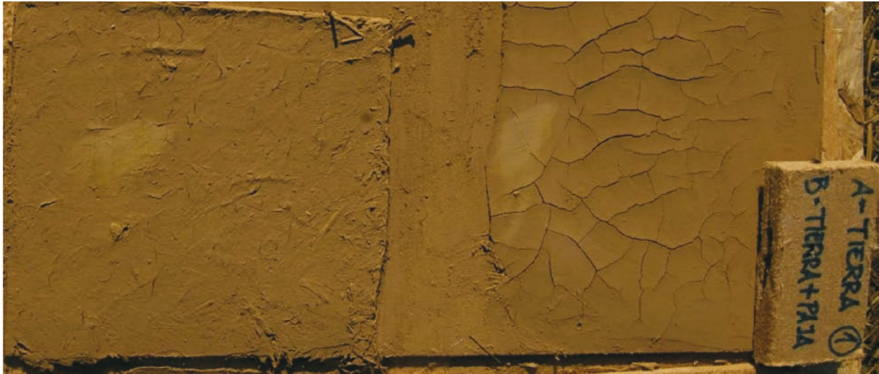
Fig. 40. Experimentation with plaster mixes. The mix on the right has cracked because of the power of the clay to pull together. The mix on the left has the same amount of clay but it has been reinforced with straw. Straw counteracts the contracting of the clay and thus prevents cracking, 2021; photo by the author
