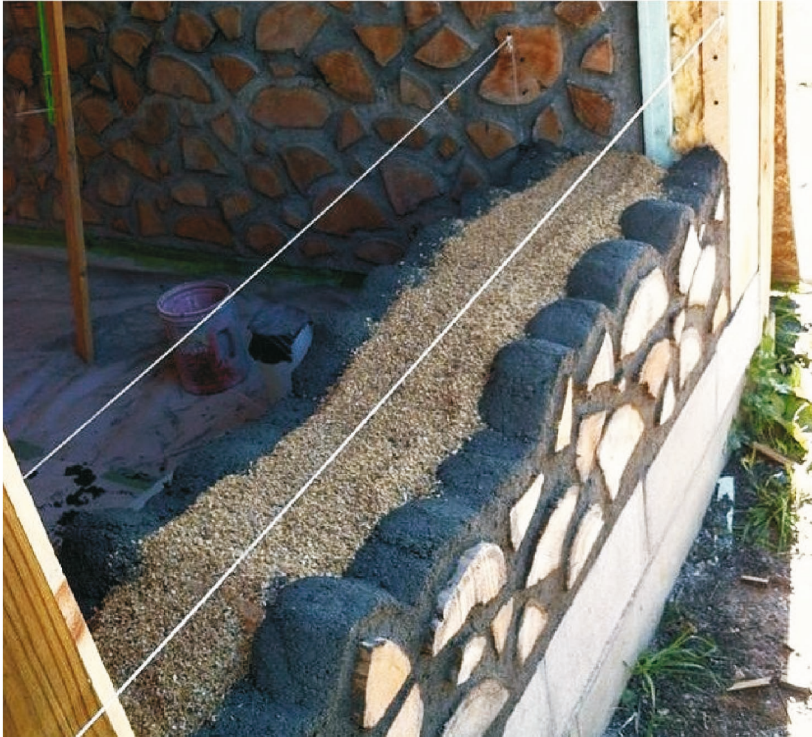
Fig. 12. Mortar is not being used along the entire length of the logs, so that a free space is made in the center. This is filled with insulation, here sawdust; photo by: [Flatau, n.d.d].
