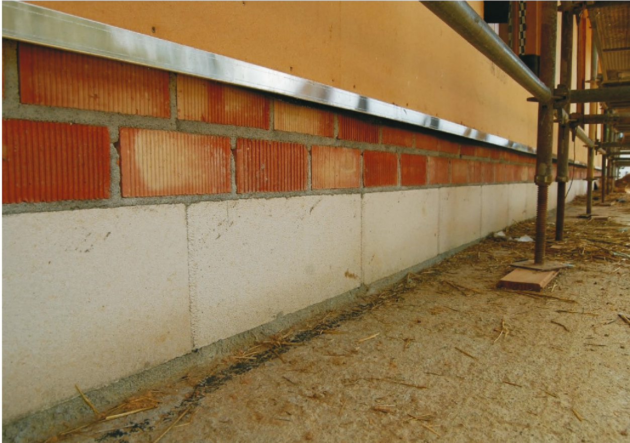
Fig. 43. The outside of a straw bale house, showing a sufficient height from the ground level of the sole of Portland cement. There is first a sole of Portland cement, then blocks and finally bricks. There is an impermeable membrane laid on top of the bricks, 2021; photo by the author
