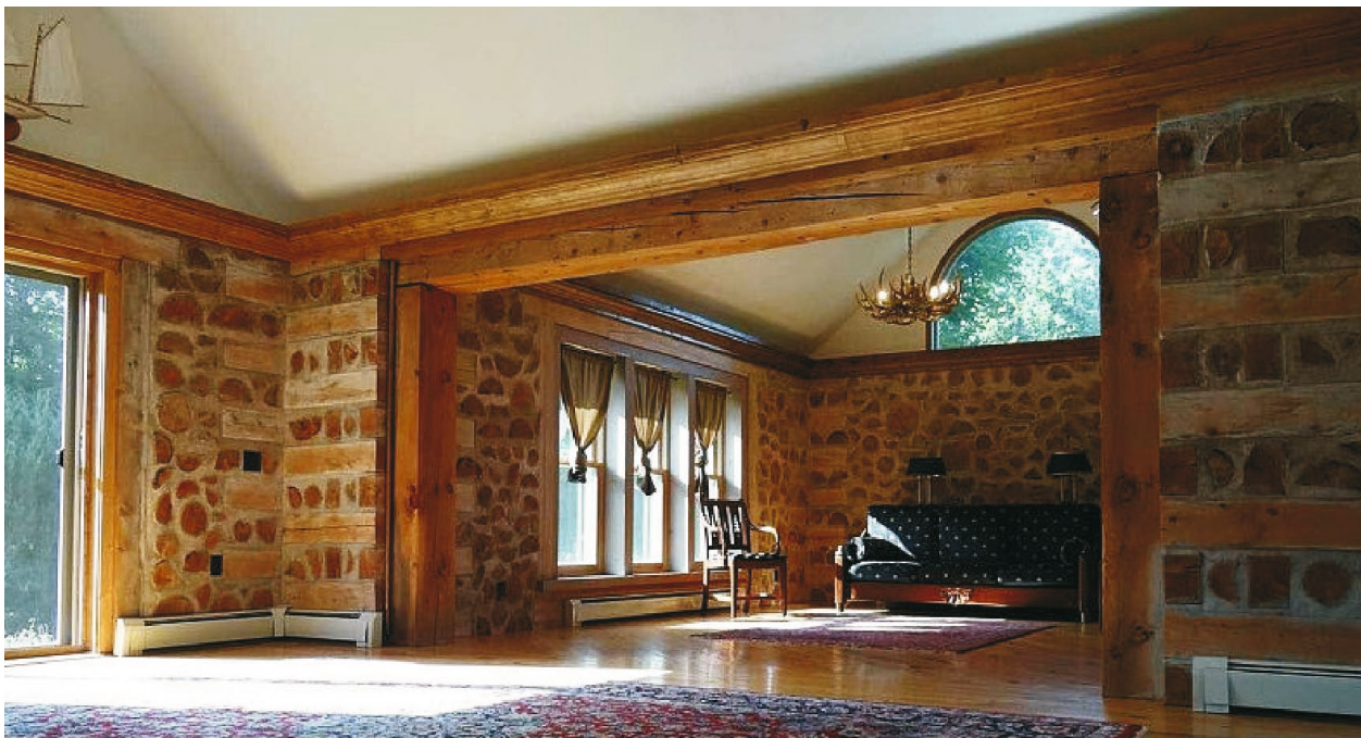
Fig. 29. Example of Lomax Corner type for anchoring also the internal corners (the nearer corner to the left in the picture); photo by: [Flatau, n.d.].
