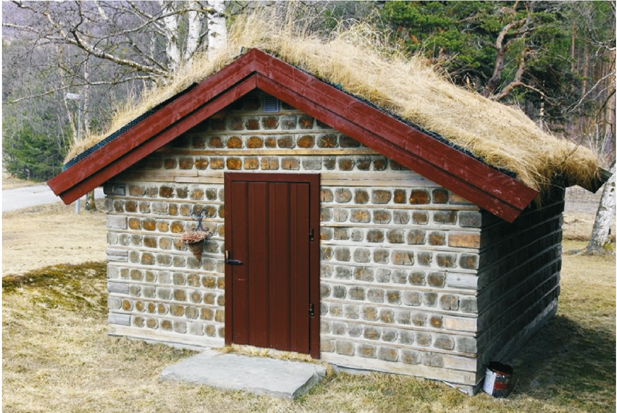
Fig. 19. A cordwood construction set up in Norway in 2008. The logs are reused wood from an older log house ( lafteverk 2 ) that had to be demolished. It is based on the historical cordwood construction technique in Norway. There are horizontal battens in between each layer of logs. The corners have logs placed on top of each other in an overlapping pattern of 90 degrees; photo by: [Stenby, 2021].
