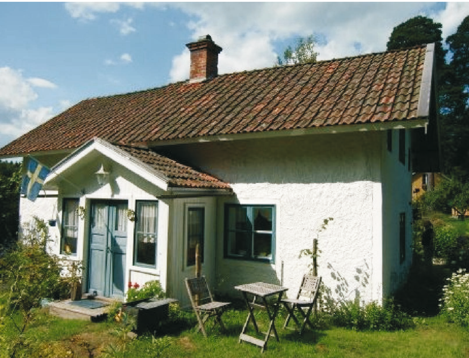
Fig. 14. This cordwood house stands in Sweden. It was built in the 1870s or 1880s. It is clad with clay based plaster; photo by: [Hagman, 2016].
