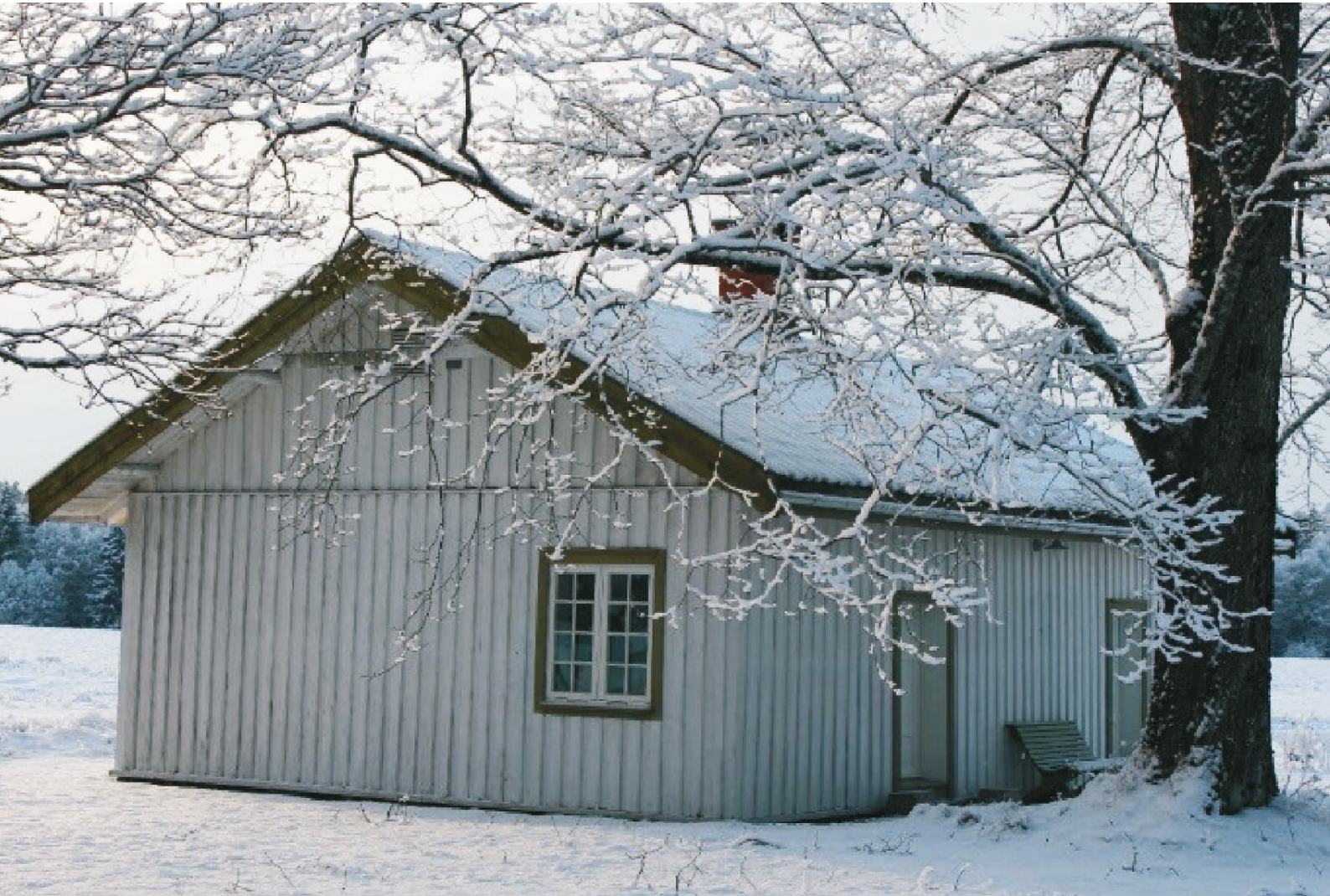
Fig. 15. A cordwood house located at Veset farm in Norway. It was built in the last part of the 1800s and is in use today as a house for living. It is clad with wooden boards like a regular Norwegian house. The cordwood wall can be seen in Fig. 16 and Fig. 17; photo by: [Nordbye, 2016].
