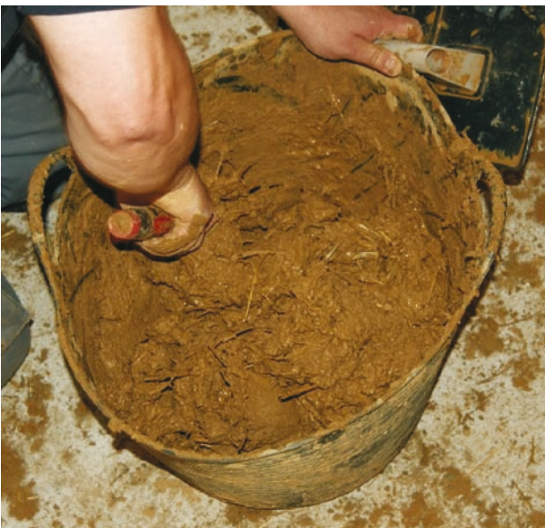
Fig. 38. Clay and straw mix being made, 2021; photo by the author
