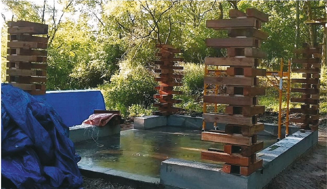
Fig. 28. An example of Lomax Corner for securing corners. The units have one less batten in height than in the example in the black and white pictures designated Fig. 25, 26 and 27. They also have a central opening. This is the individual project variation; photo by: [Cordwood Construction, 2019].
