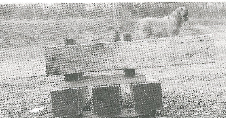
Fig. 25, 26 and 27. An overview of a type of a Lomax Corner unit to see the design and how they are stacked. The dimensions of the beams in thickness and length can be different for different projects, photos by: [Roy, 2003, p. 46]
