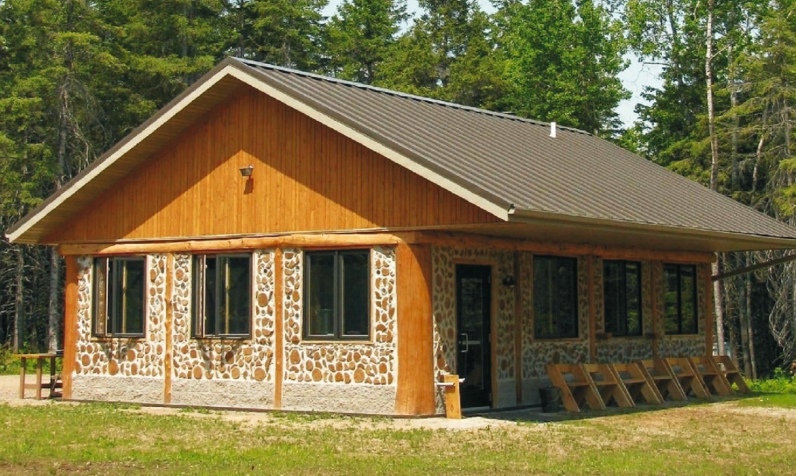
Fig. 44. Cordwood house with large roof overhangs so that rain will not hit the mortar directly in any place. (There can also be seen a good ringwall up from the ground); photo by: [Flatau, n.d.].
