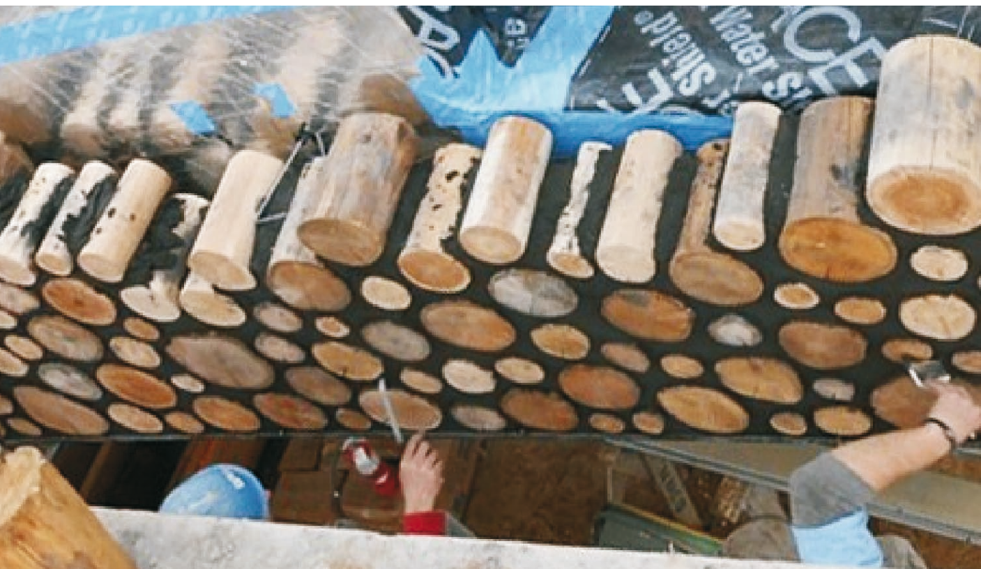
Fig. 11. Construction technique of cordwood masonry in its most basic form; photo by: [Kalamazoo College, 2014].
