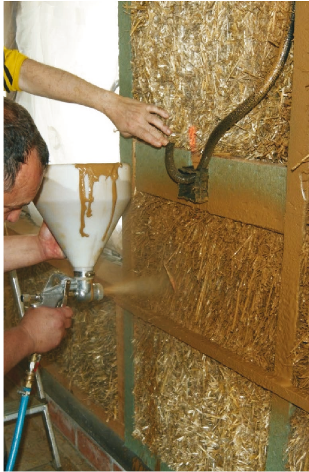
Fig. 37. Spraying on the clay-water mix. In this case it is on straw bale but it serves as an example, 2021; photo by the author
