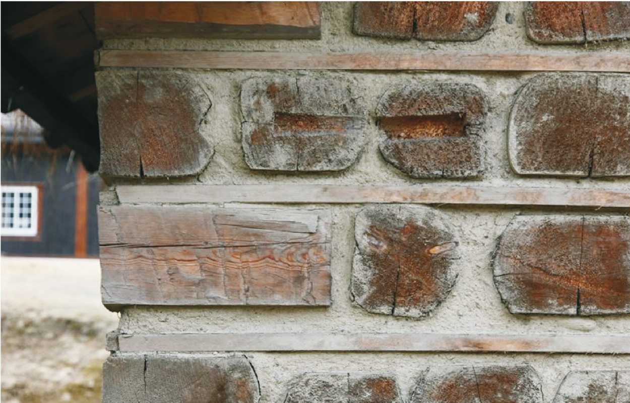
Fig. 21. Closeup of the corner of the 2008-construction in Norway in Fig. 19. The corners have logs placed on top of each other in an overlapping pattern of 90 degrees. There are battens in between each layer of logs. There is always a part of mortar separating the parts of wood; photo by: [Stenby, 2021].
