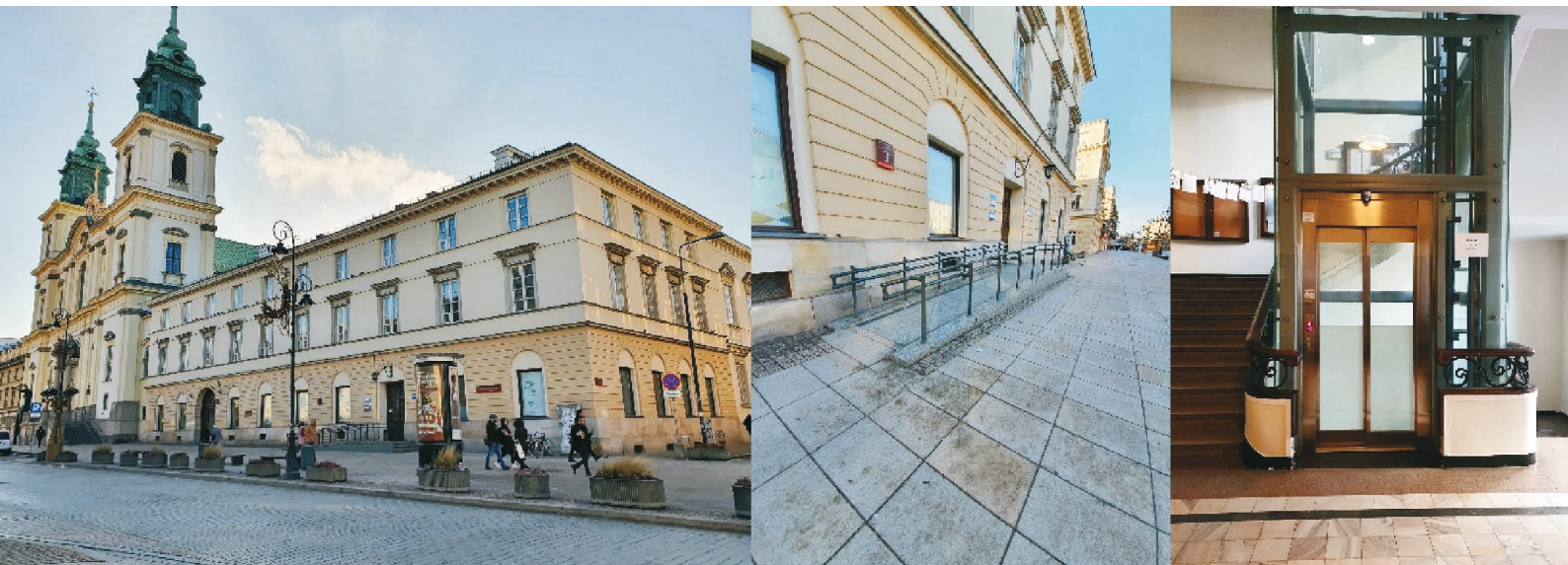
Fig. 3. University of Warsaw, Institute of Philosophy – ramp for persons with disabilities, interior lift; source: photo by the authors
