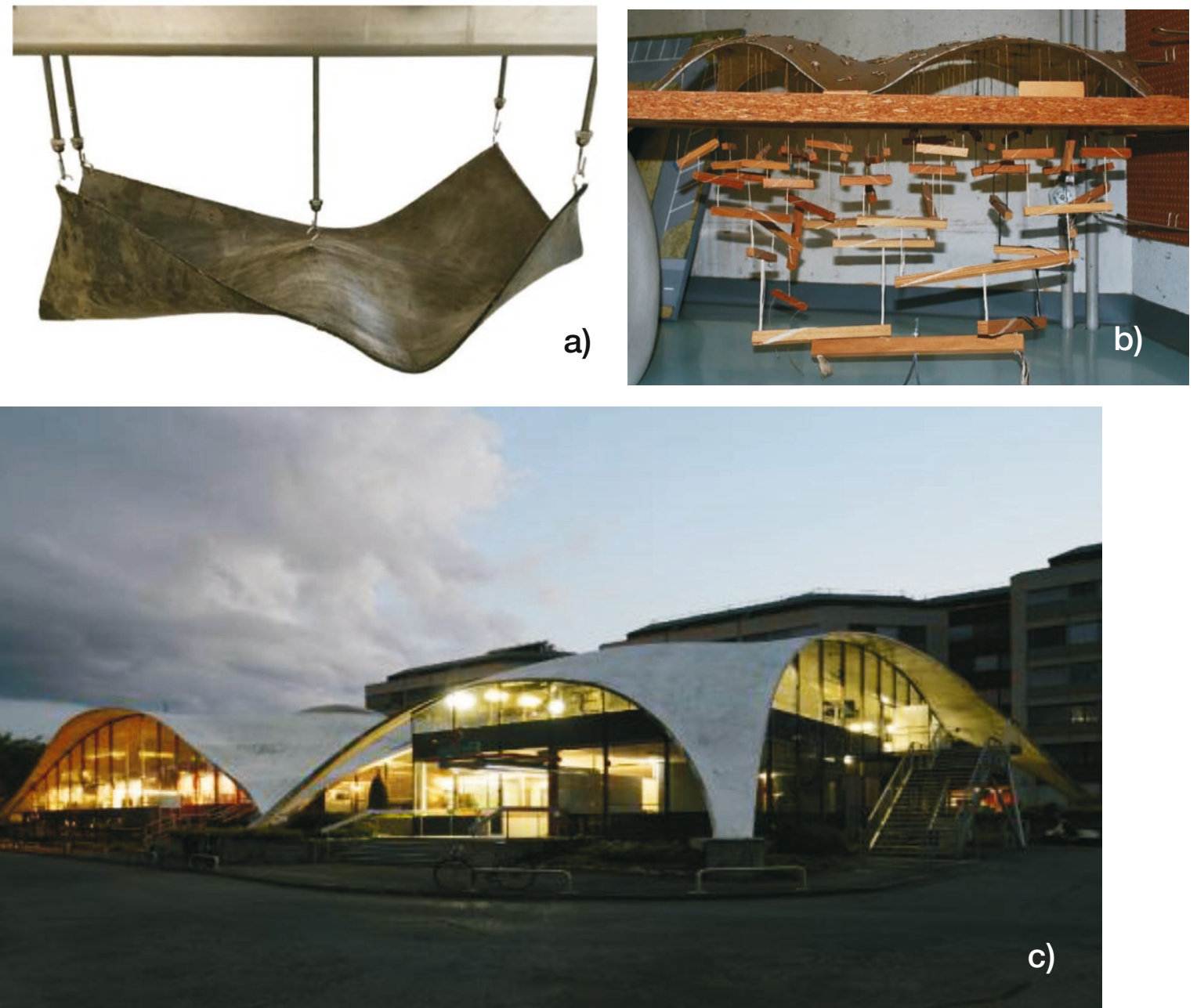
Fig. 3a-c. Heinz Isler, Sici SA Factory in Geneva, 1968–1969, a) elastic rubber model small-scale epoxy resin model, b) the model used for the evaluation of structural behavior of the Sici SA Factory in Geneva, c) Sici SA Factory in Geneva; source: J. Chilton (2011); C.C. Chuang, J. Chilton (2016)
