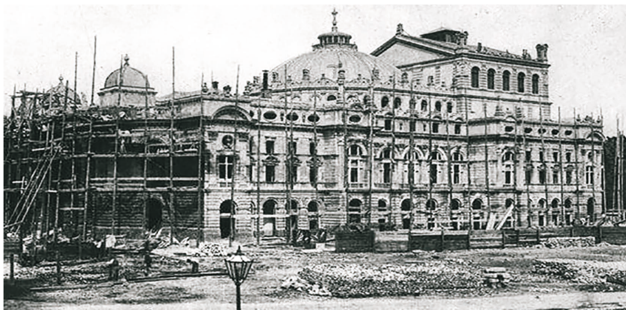
Fig. 3. Slowacki Theatre construction, Krakow 1891, Slowacki Theatre Archive; source: www.https://teatrkrakowie.pl/poczatki
