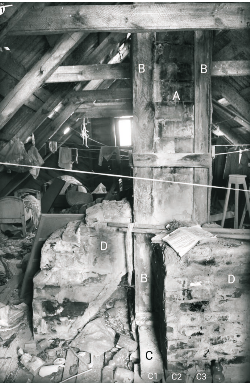
Fig. 11. The attic with the longest smoke flue (C) exposed; photos by the authors, 2018
