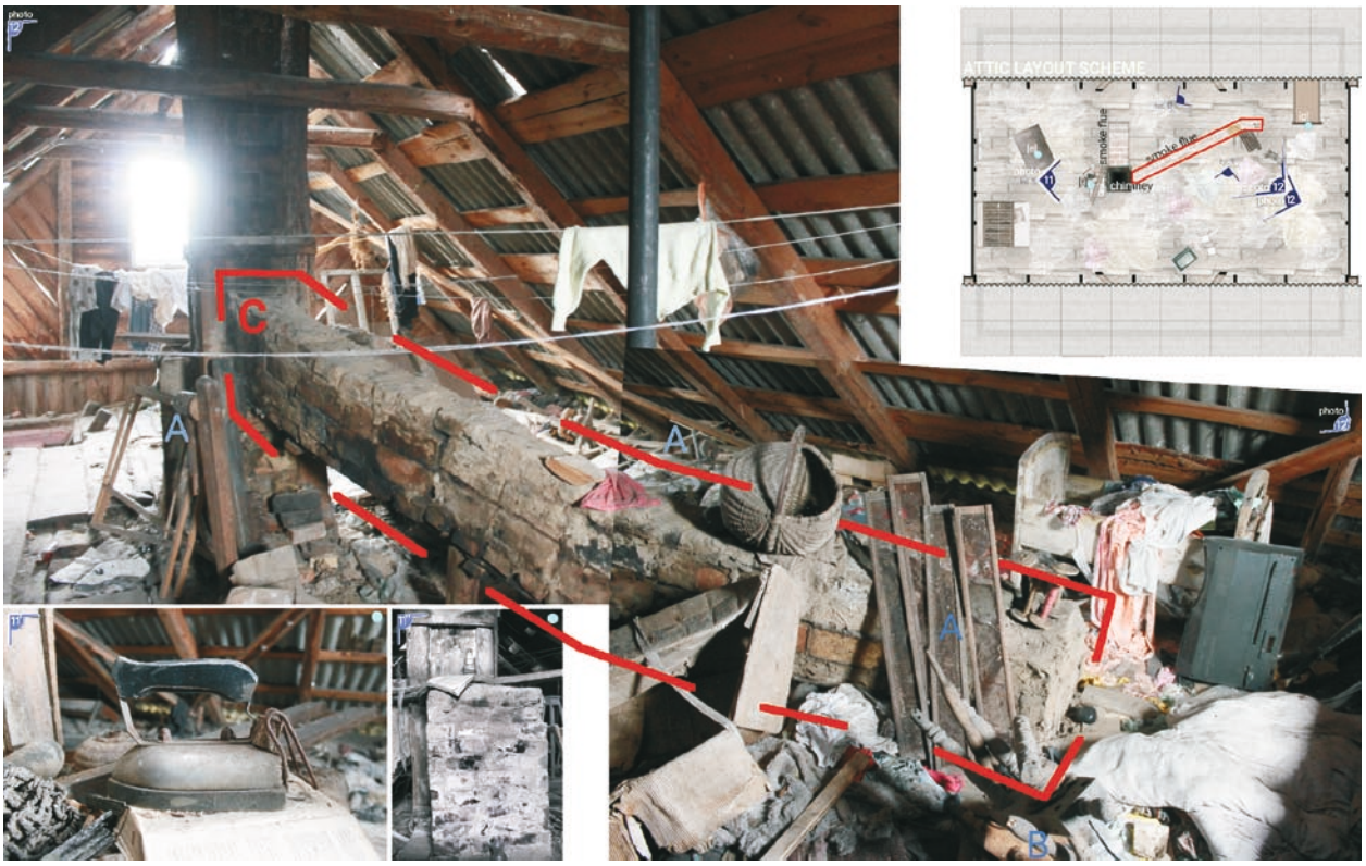
Fig. 11. The attic with the longest smoke flue (C) exposed; photos by the authors, 2018
