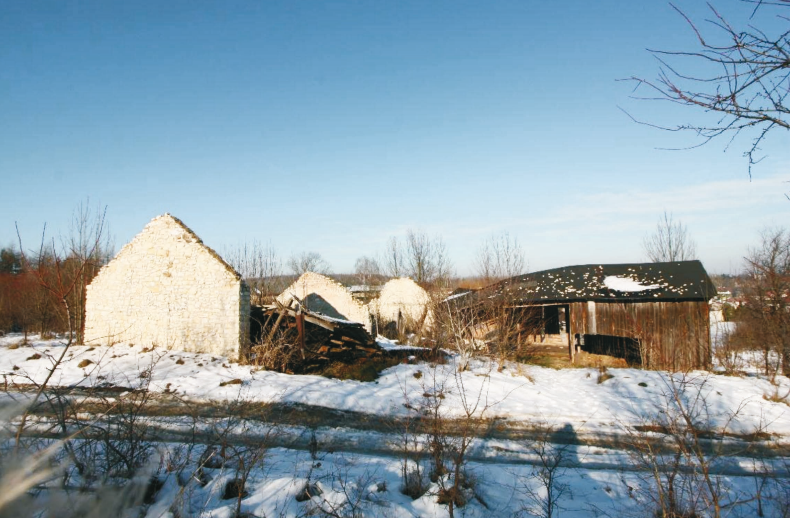
Fig. 7. Current condition of the barn complex in Mstów. The photograph shows the stone gable walls of Barn No. 1 and Barn No. 2 (with a shared central wall). On the right side, Barn No. 3 with its timber structure visible. The buildings are in a state of ruin; source: photo: Andrzej Kos, February 2025.
