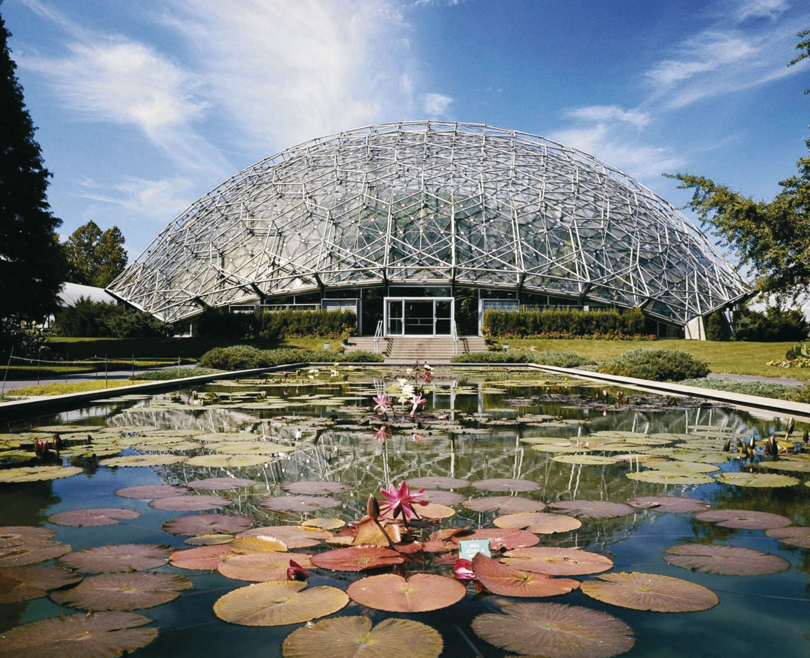
Fig. 5. Buckminster Fuller, Climatron. Geodesic Dome, Missouri Botanical Garden, St. Louis, USA, 1959; source: [N. Paszkowska-Kaczmarek 2022]
